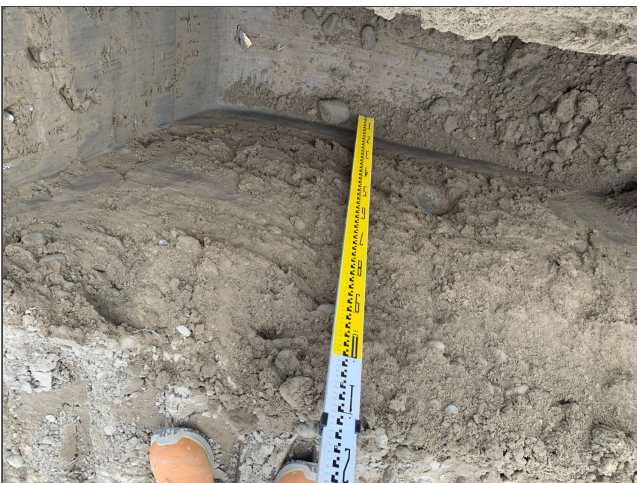
Fig 3. TP02 - fill/silt contact at 0.8 m.
