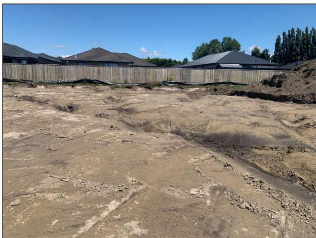
Fig 1. Overview of Lots 152 and 153, facing SW. All Topsoil and unsuitable material have been removed to natural ground before inspection.
