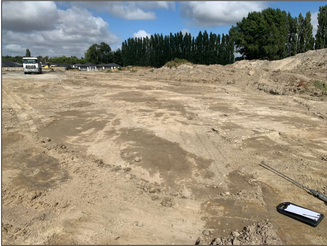
Fig 4. Overview of ROW1, facing SW. topsoil and unsuitable materials was stripped prior to arrival.
