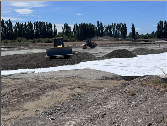
Fig 4. Basal filter cloth installation. Note some hollows were filled prior to cloth placement.
