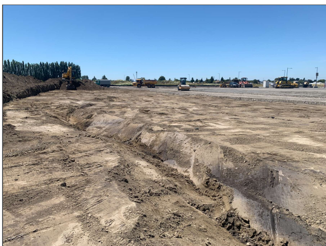
Fig 2. Overview of Lot 154 to 158 facing NE. Topsoil and unsuitable material have been striped before inspection.
