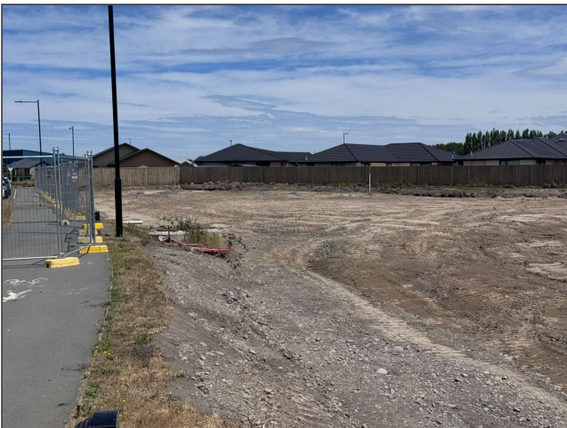
Fig 8. Previous settlement monitoring pad on elevated area comprising lots 187-190. DCP testing indicates this is engineered fill from previous works.
