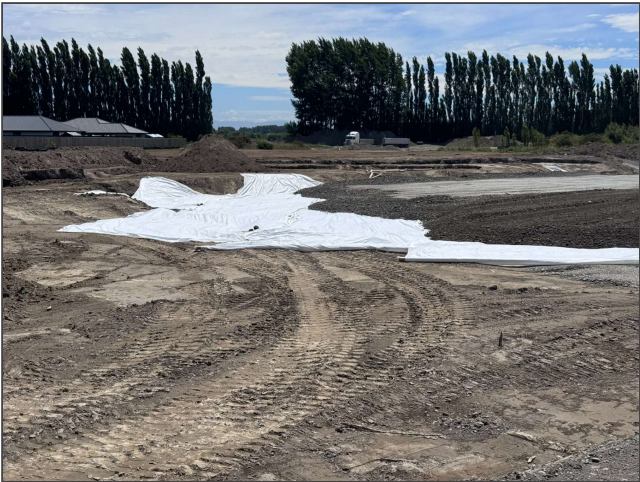
Fig 3. site overview from south boundary showing earthworks placement over previously inspected lots 169-177
