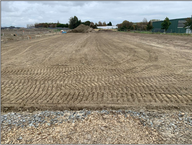
Fig 1. Looking from NE corner of site westwards across Lots 123-117. Stockpile in Background is on Lot 117. In February 2026 this was a stormwater retention pond. It has now been backfilled with gravelly silt/fine sand.
