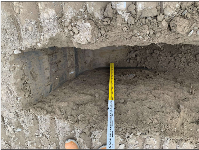
Fig 4. TP03 - fill/silt contact at 0.9 m
