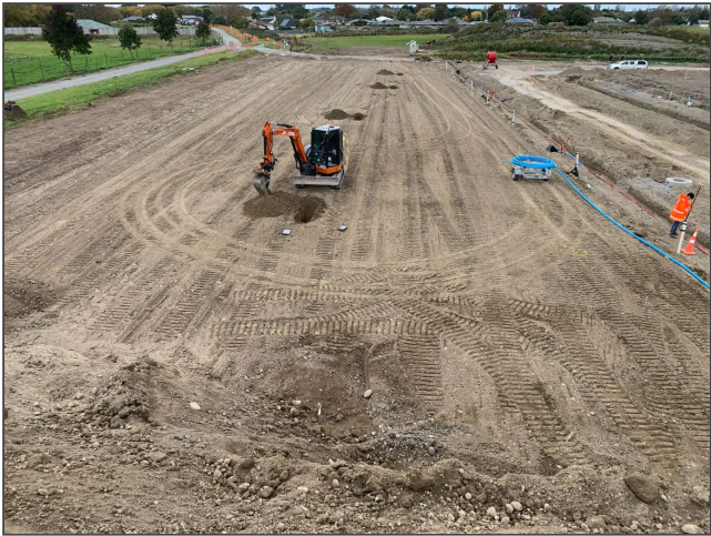
Fig 6. Photo from top of stockpile showing test pit locations from TP01 in background to TP04 in foreground.
