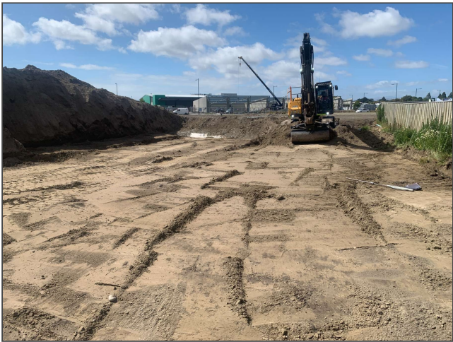
Fig 6. Overview of partially stripped Lot 164.
